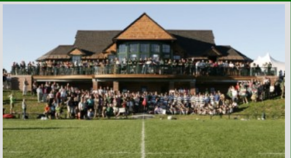
The new Corey Ford Rugby Clubhouse at Dartmouth
